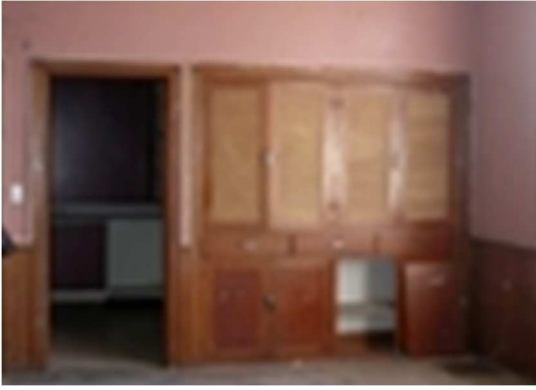
Bookcase restored and replica hardware added (We would still like to restore the glass to include the original panes)
