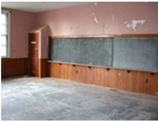
Floor sanded, a piece of slate added and a replica piece added in blackboard. (would like artist to finish it to be a closer replica) Wood floor sanded and varnished. All wood restored and antique brass hardware added to doors since there was not any hardware existing.
