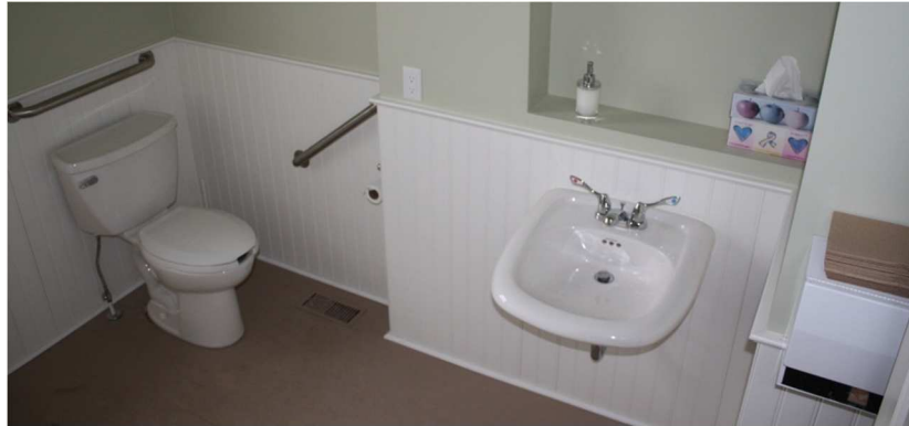
Bathroom expanded to be accessible, new sink and toilet, new solid wood door, floorboards replaced where we found sheets of plywood to match existing wood floor. New solid wood door added to match existing doors in schoolhouse.
